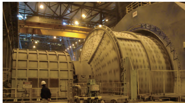
Copper concentrates processing plant at the Caserones Copper Mine
