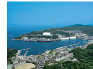
Saganoseki Smelter & Refinery, JX Metals Smelting Co., Ltd.
