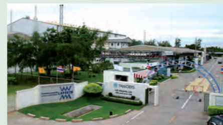
TANIOBIS's Thailand plant
