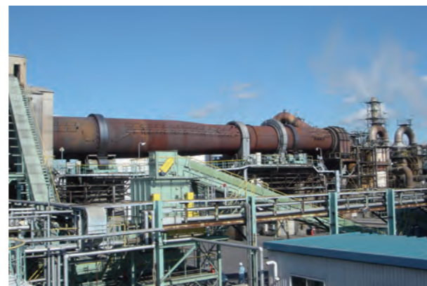
Rotary kiln incinerator at JX Nippon Tomakomai Chemical Co., Ltd.
